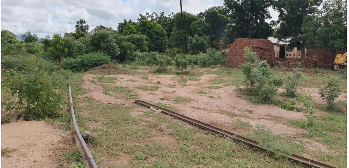
*Above and Below: Around 60% of the rail sleepers on the 76km of line from the border at Marka to Bangula have been stolen, and 15% of the rail has been removed. The rail from Nsanje to the Mozambican border last ran in 1983, and from Nsanje to Bangula in 1996. The cost of rehabilitation ranges from \$750,000 per km for basic refurbishment of the permanent way, to \$3 million for more extreme reconstruction.*
