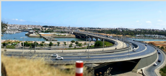
Bridging the gap: The 1.2 km-long Hassan II Bridge brings Rabat and Salé closer together
